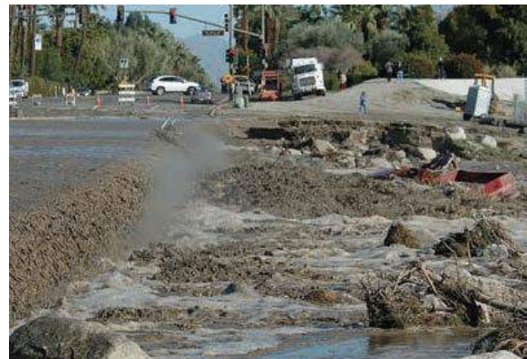
CVWD's Stormwater Facilities Provide Flood Protection
