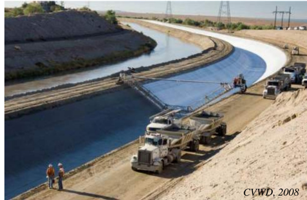
Coachella Canal lining project
