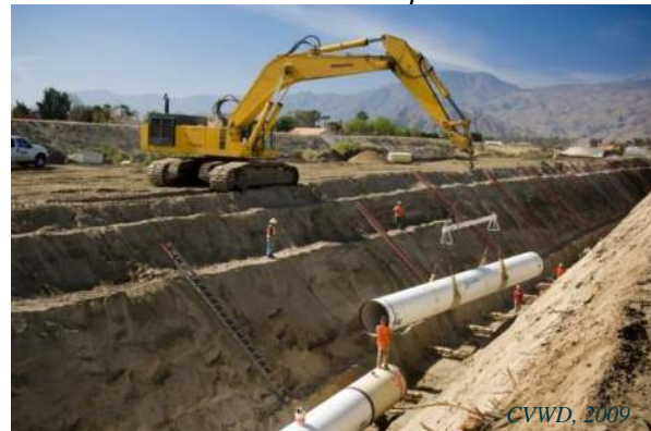
Installation of 54-inch Mid-Valley Pipeline for delivering recycled water
